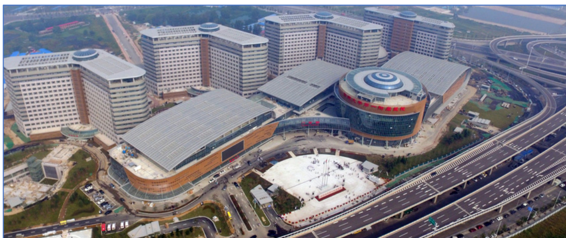
Hospital in China
